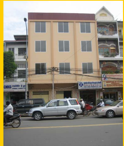
Building 2 located along Street 128 (Kampuchea Krom Blvd)
